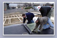
To waterproof elevated slabs, select from a versatile range of asphaltic membranes: hot melt PENNCOAT™ 101 Membrane, cold-applied TUFCHEM II Membrane, or adhesively bonded PENNCOAT 600 Membrane sheet.
